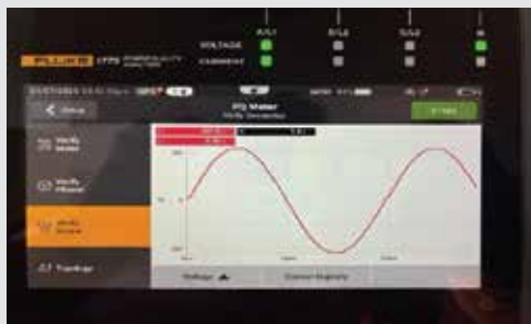
Power waveform of any conventional UPS for radiology equipment during peak processing
